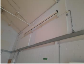
4.5 metre wide screen fixed to the wall on four special TSPProfessional brackets
