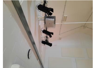
Video projector and new lighting bar fixed using a special wall bracket with security cage
